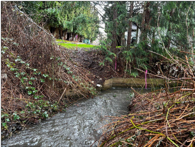
Photo 9: Southeast slope conditions to the south of subject parcel. Note pipes directing to creek.
