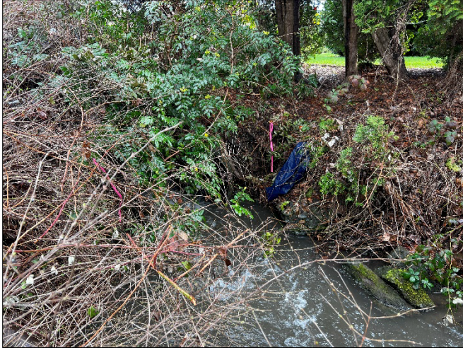
Photo 7: Creek exiting culvert along NE corner of site.
