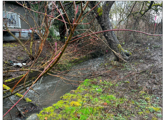
Photo 10: Southern boundary of site. Grades are generally steeper out of site. Note lagging along southern slope.
